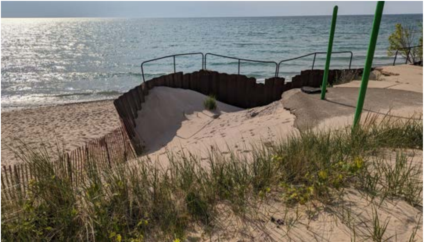
Image 1: Existing Sheet Pile Wall
